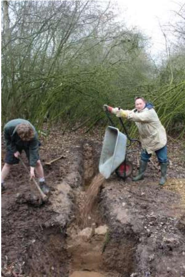
A composting toilet is being installed, to improve facilities for schools and groups, wishing to use the site. Due to the impervious clay substrate, a soakaway has been added, to keep the main chamber dry and stop it becoming anaerobic and smelly.
